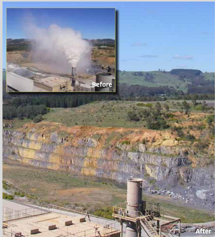
Dust control on the kiln stack at Railton was previously handled by two precipitators installed in 1965 and 1980. The precipitators were no longer able to meet the required standard for dust emissions. Both precipitators were replaced by a single modern bag filter.
